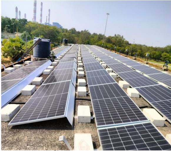
1) Stadium gallery – 40 KWp
