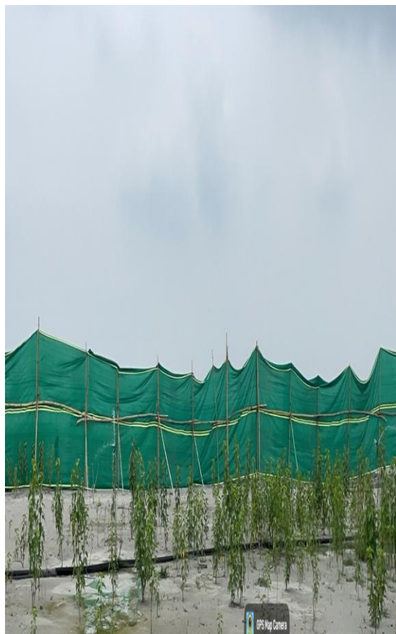
Shade net/Agro mesh Installation.
