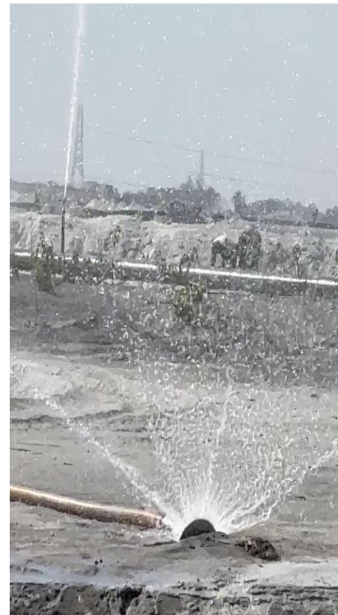
Installation of Water curtain.
