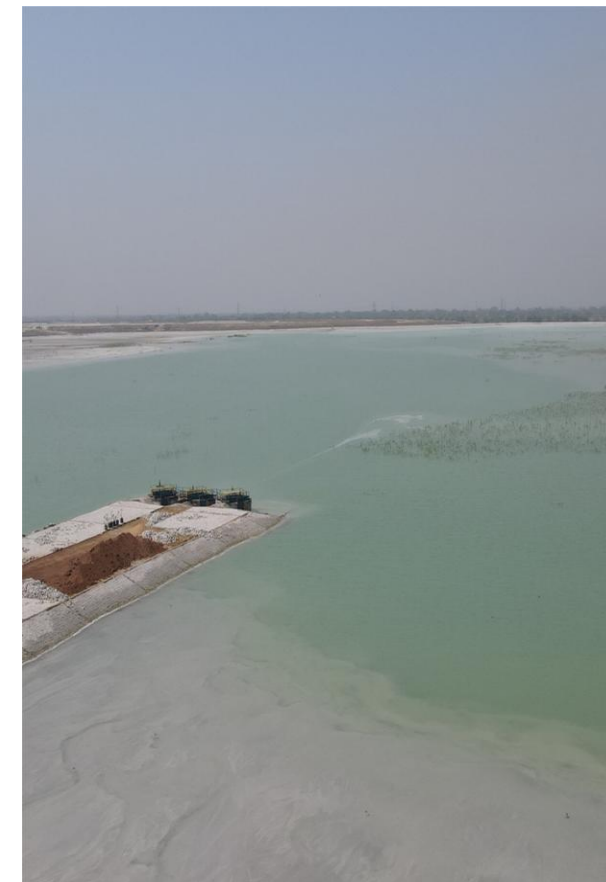
Ponding of charged Ash dyke
