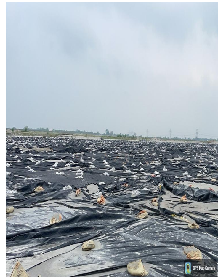
Laying of Tarpaulin Sheet.
