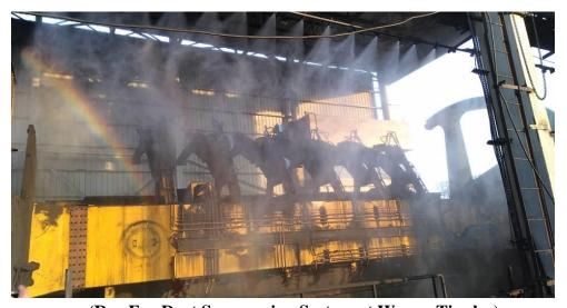
(Dry Fog Dust Suppression System at Wagon Tippler)
