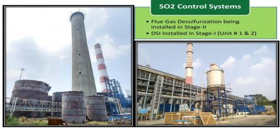
Flue Gas Desulphurization and Dry Sorbent Injection System for SO2 Control
