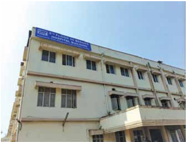
50-bedded Hospital building in Telangana
