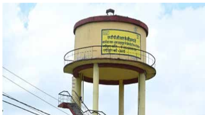
Overhead Tank in village Armuda (Lara)
