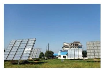
53 Kw Concentrated Photovoltaics Module setup, NETRA
