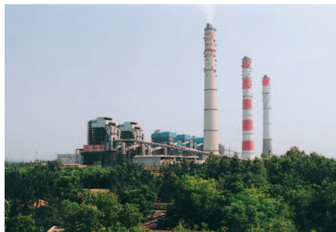
A panoramic view of Talcher Project
