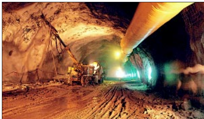
Tunnel work nearing completion at Koldam
