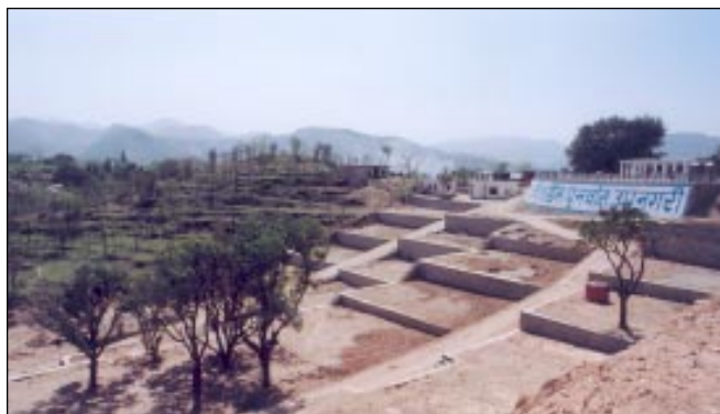
R & R Township under construction at Koldam
